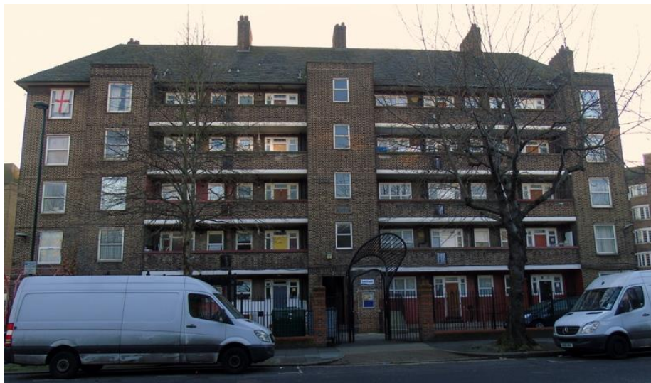
Flats on the Briant Estate in Lambeth
