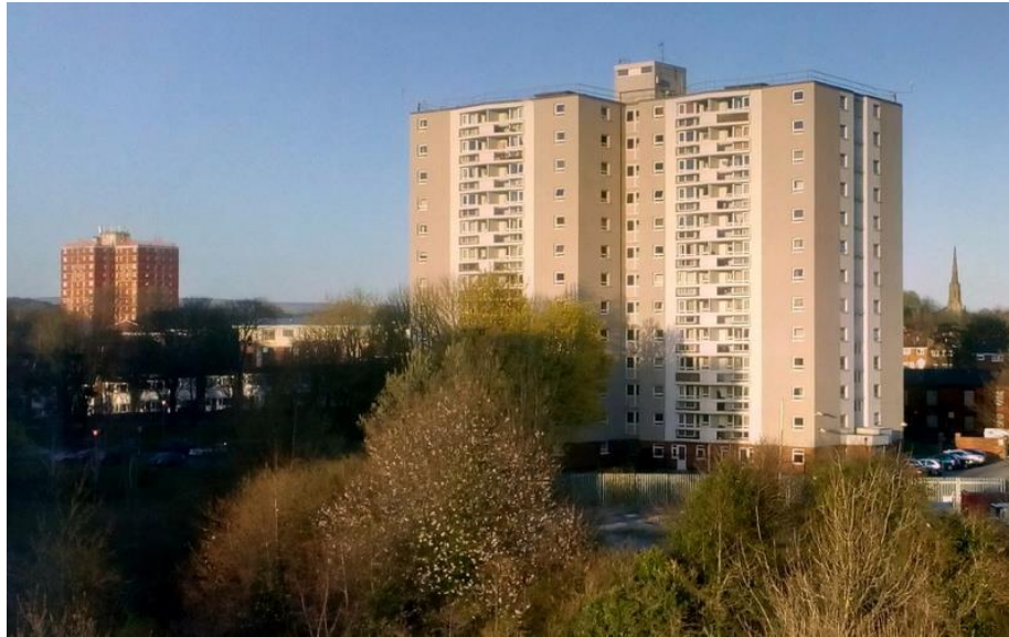
Council Flats in Wigan, Greater Manchester
