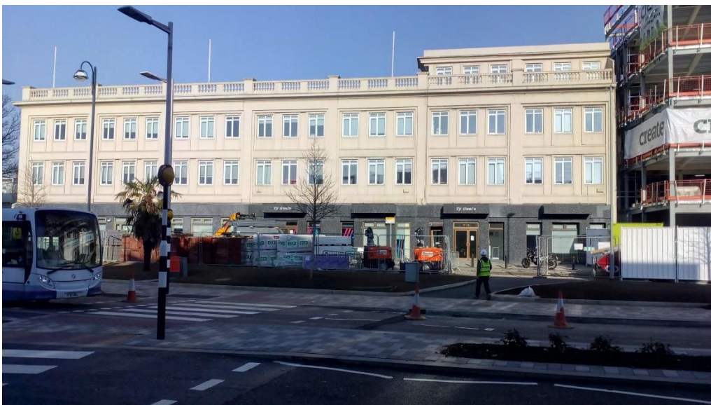
The offices of POBL Housing Association in Swansea.
