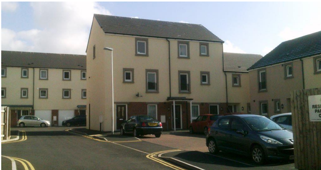
Ridley Court, a development in Penrith, Cumbria, by Impact Housing Association.
