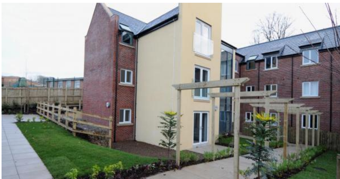
Bramble Court, an Impact Housing Association Extra Care Elderly scheme at Brampton in Cumbria
