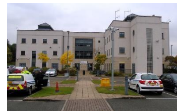
Denbighshire County Council Offices in Denbigh. Denbighshire Council has retained its housing stock.
