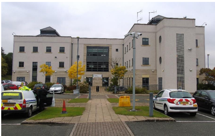
Denbighshire Council offices in Denbigh. The Council has just completed a consultation on its Homelessness policies.
