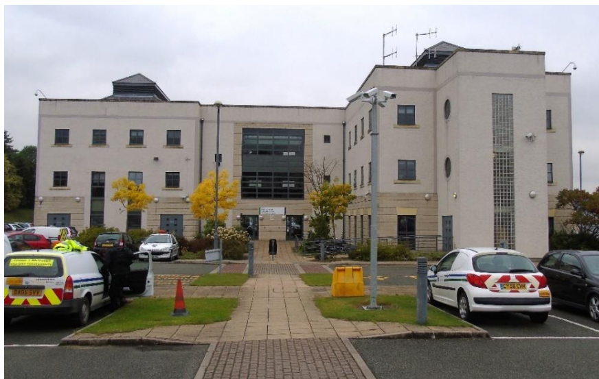
The offices of Denbighshire County Council in Denbigh. The Council un-pooled service charges in 2015.
