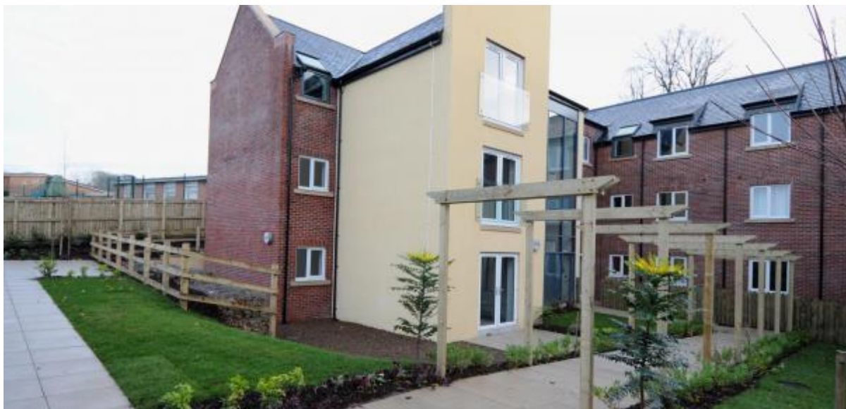
Bramble Court, Brampton, Cumbria. An extra care elderly scheme opened recently by Impact Housing Association. Such schemes are now threatened by proposed changes to their funding.
