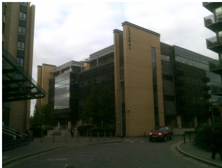
The offices of the Homes & Communities Agency in Leeds.
