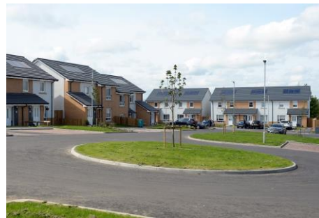
New Council Houses in North Lanarkshire
