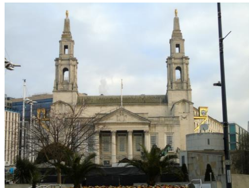
Leeds Civic Hall
