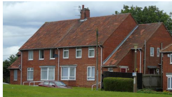
Council Houses in Gateshead, Tyne & Wear.
