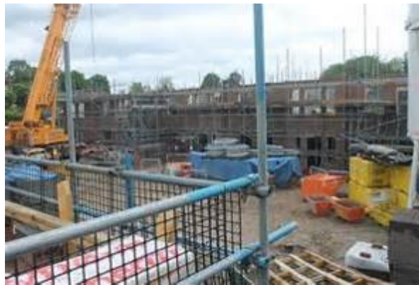
New Council Homes being built in Ashfield, Nottinghamshire.
