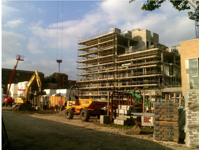
New Homes being constructed by Catalyst Housing Association in Kensington, London.
