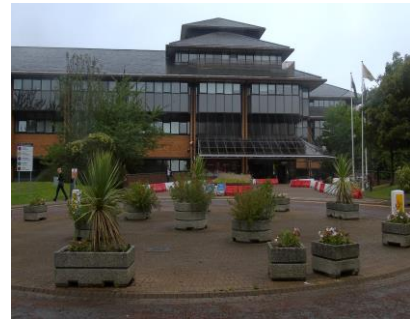
County Hall at Cardiff. Cardiff City Council is one of the largest landlords in Wales.
